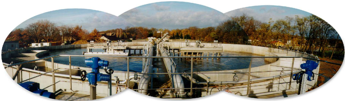
Figure 8. CYCLAZUR™ Cyclic activated sludge technology at WWTP Potsdam
