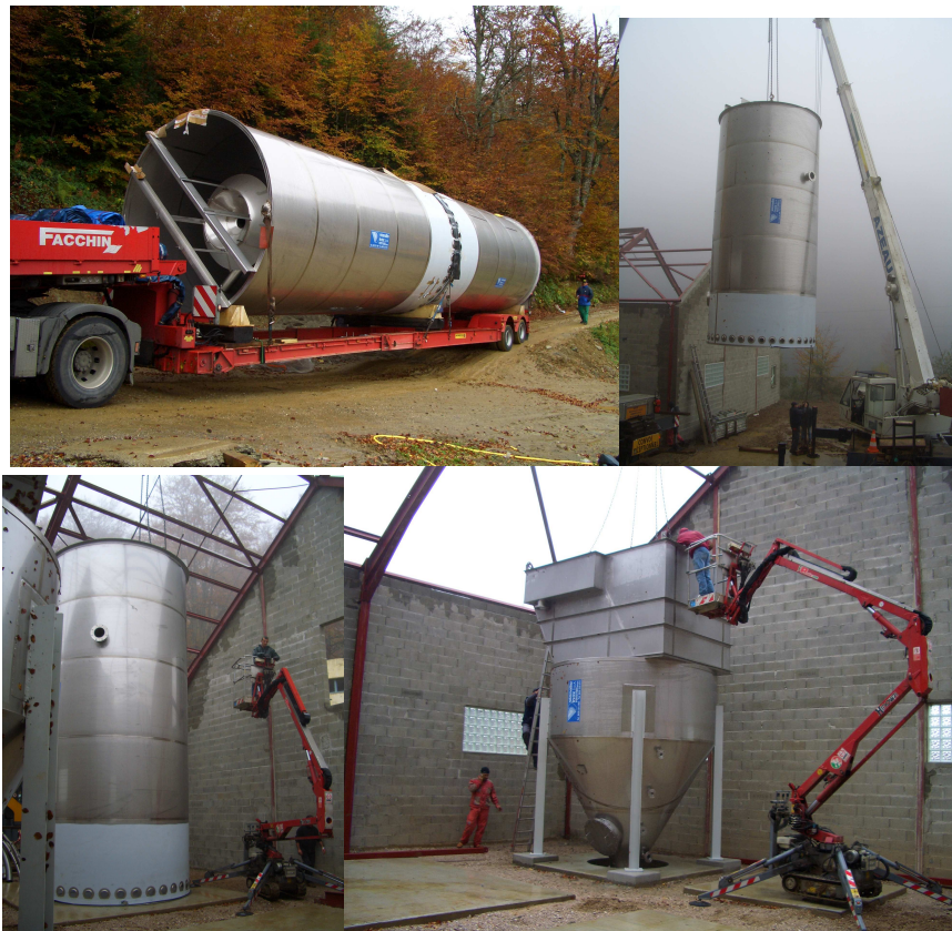
Figure 4: Delivery and mounting of BAF filter and lamellar clarifier
